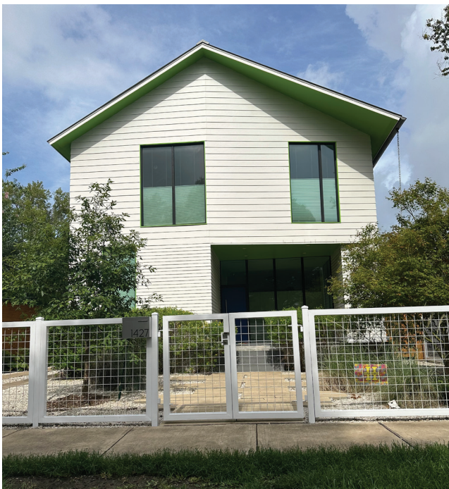
1427 Allston St (built in 2019) - Houston Heights East Historic District (Non-Contributing)
